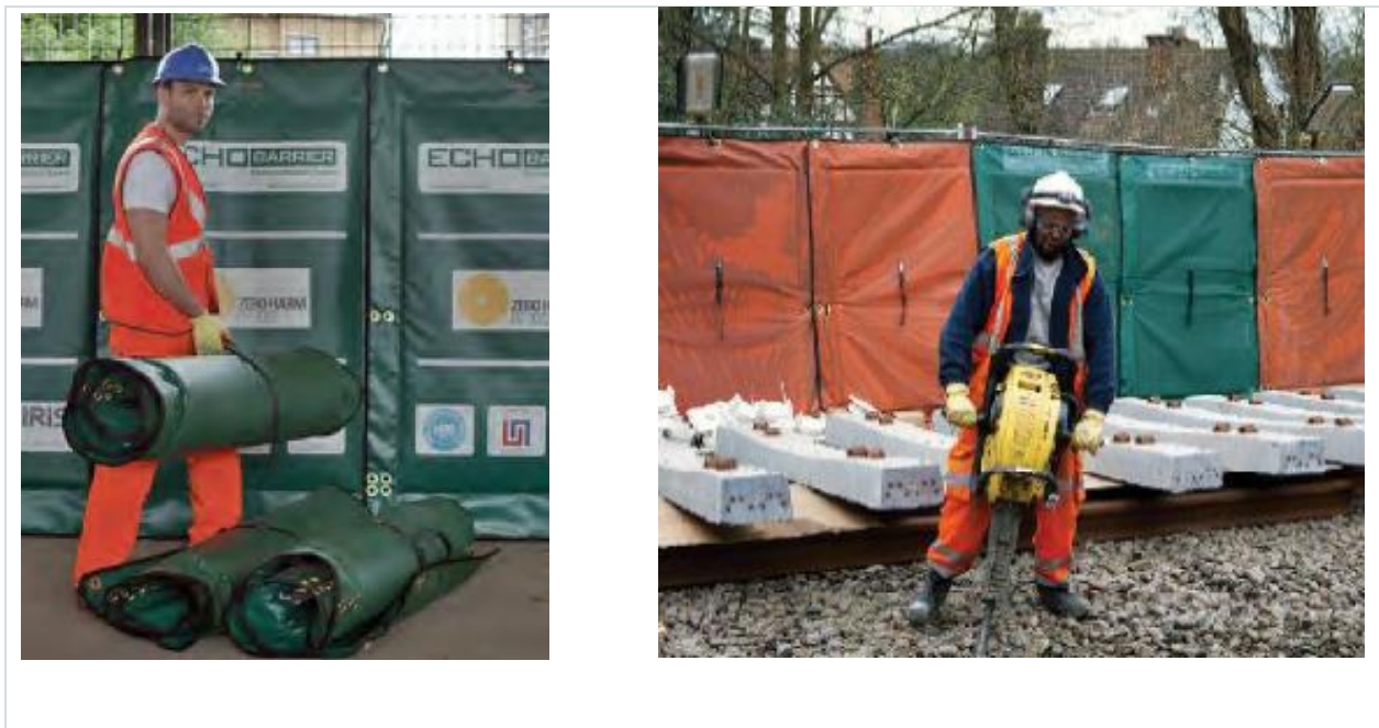
Figure 4: Photos of demountable noise barriers
